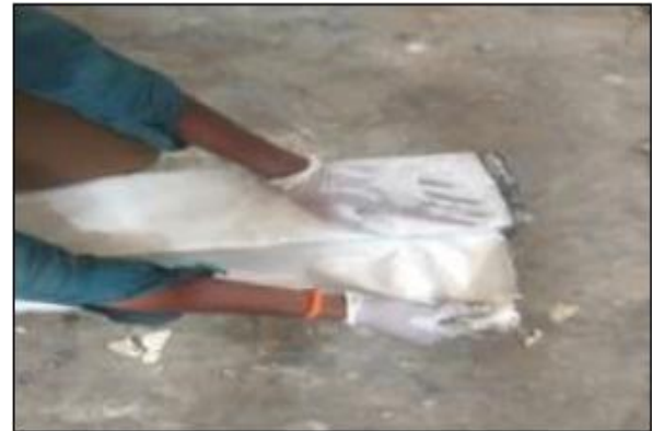
Fig. 4: Applying Glass Fiber Sheet on Beams
