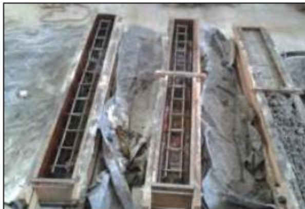
Fig. 2: Casting of Beams
