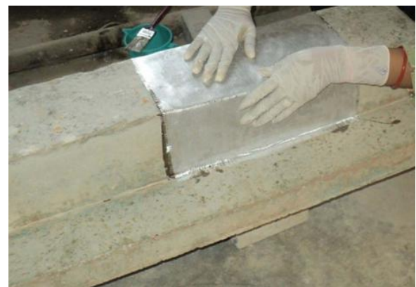
Fig.4.3. Fixing of GFRP sheets on the beam.
