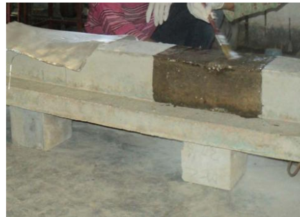
Fig.4.2. Application of epoxy and hardener on the beam
