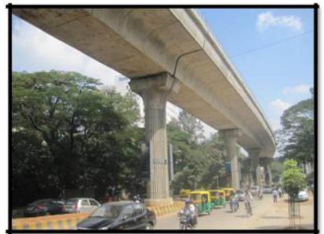
Fig.1.1. Typical Elevated Metro Bridge.
