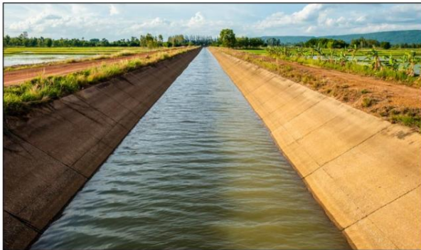
Figure: Irrigation canal
